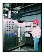
Colts MAXIM RTO systems are provided with Allen-Bradley programmable logic controllers, and Honeywell burner controllers as standard equipment. As a trend today, many of our systems have been provided with a network interface, to allow monitoring and control of the MAXIM RTO from remote locations - on or off the plant site.
