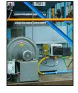
Combustion air blowers are provided with inlet silencers and air filters to minimize ambient noise, and protect the blower from dust and particulates.
